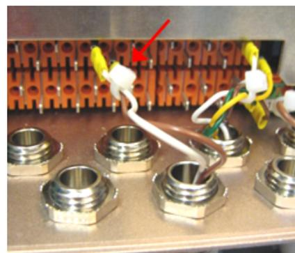
9. Cut the cable tie as near as possible to the wires.
