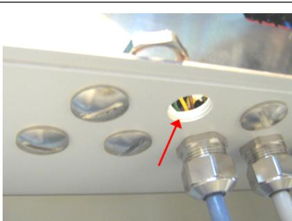
1. Select an unused opening nearest to the cable connection on the electronic board. Remove the screw and nut combination and set aside the screw for later use.
