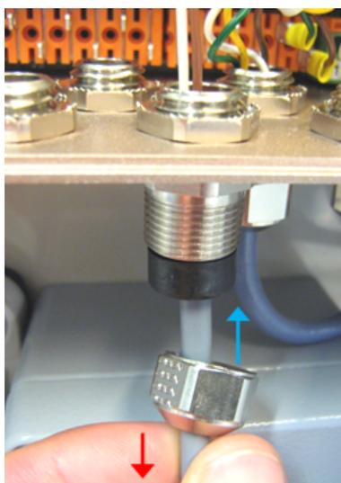
5. Pull the cable slightly with one hand until the inner shield comes into contact with the gland. Tighten the nut onto the gland with the other hand.
